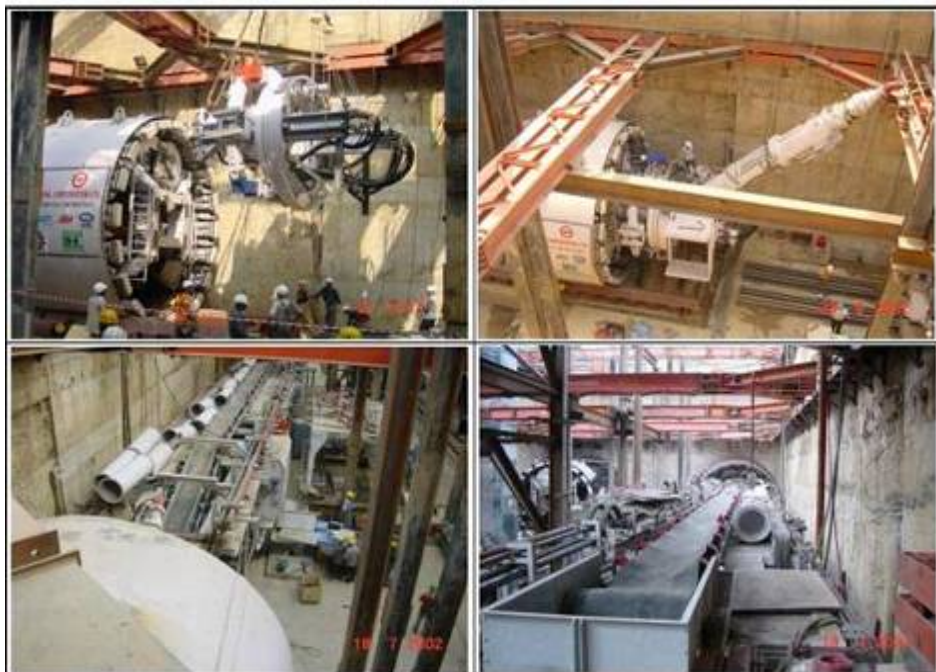
Figure 4.16: Erector, Screw Conveyor & Backup System
