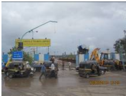
1. Construction at the site of proposed metro station
