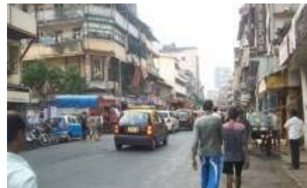
2. Insufficient width of footpath results in pedestrian movement on carriageway
