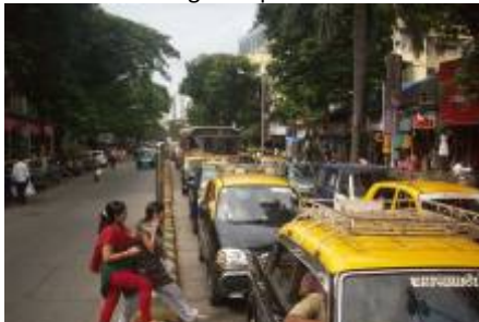
3. Pedestrian – vehicle conflict due to absence of pedestrian crossing facilities
