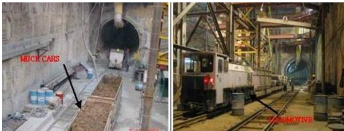
Figure 4.17: Excavation
