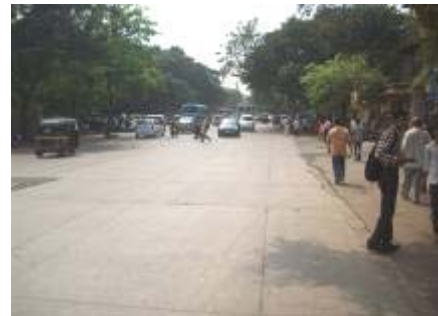
2. Pedestrian – vehicle conflict due to absence of pedestrian crossing
