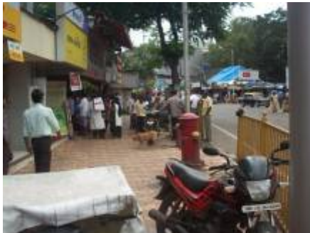
1. Encroachment and on-street parking of vehicles on footpath
