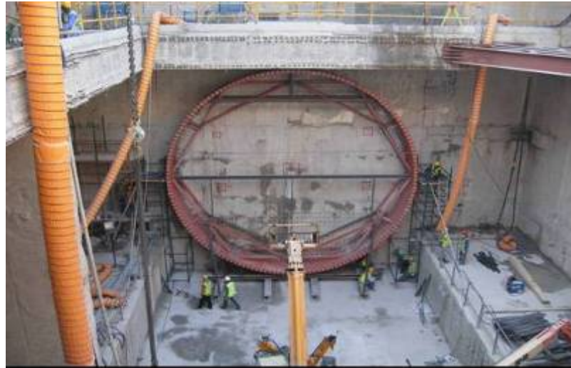
Figure 4.16: Erector, Screw Conveyor & Backup System
