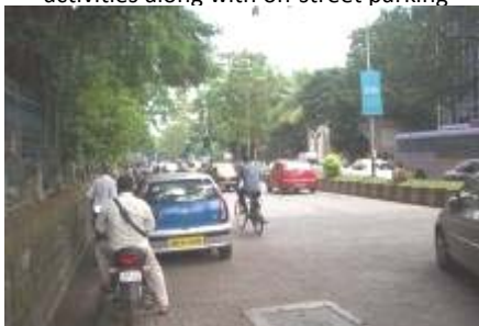
5. Absence of footpath results in pedestrian traffic conflicting with vehicular traffic
