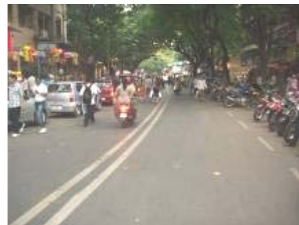
2. Pedestrian – vehicle conflict due to absence of pedestrian crossing facilities
