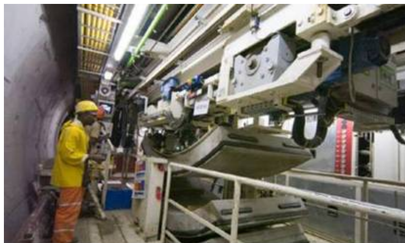
Figure 4.20: Operator Controlling the Movement of the Pre-cast Tunnel Segments
