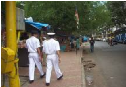
1. Encroachment on footpath obstructs the pedestrian movement
