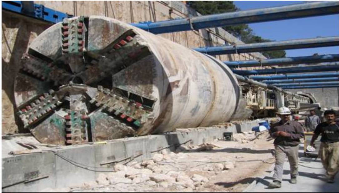
Figure 4.22: TBM pushed to the other end of the station
