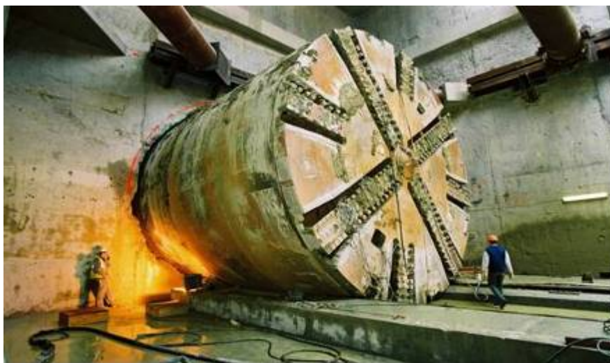
Figure 4.21: TBM through the diaphragm wall
