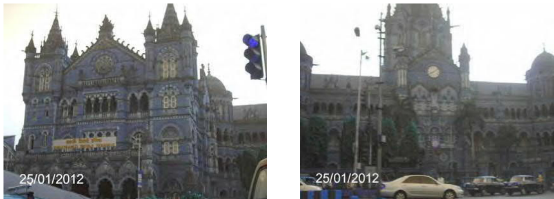
FIGUR E 3.57 PHOTOGRAPHS SHOWING CHHATRAPATI SHIVAJI TERMINUS BUILDING
