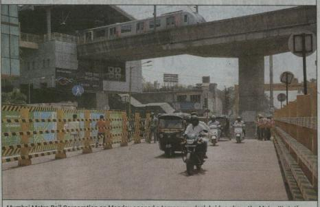
Mumbai Metro Rail Corporation on Monday opened a temporary deck bridge above the Metro III station that is being dug under Marol-Maroshi Road. The 120m long and 9m wide bridge has been erected to allow traffic movement, without affecting the Metro work. It also has a 1.5m wide pedestrian walkway. "The bridge is slightly elevated so there will be no waterlogging during monsoon," said an MMRC spokesperson
