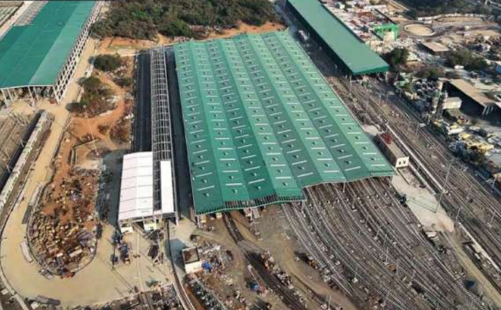
DRONE VIEW OF CARSHED
