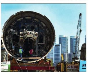
umbai Metro Rail Corporation (MM-RC) on Thursday achieved another milestone with its 28th breakthrough. from CSMT to Mumbai Central (Metro III). Vaitarna-2 is the first tunnel-boring machine (TBM) to complete 4km in one drive. The TBM was commissioned on February 2, 2018, from CSMT. by launching a shaft, and completed its longest run at Mumbai Central station with 2,730 RCC rings. "It was challenging as the alignment is close to dilapidated buildings," said MMRC MD Raniit Singh Deol. TNN
