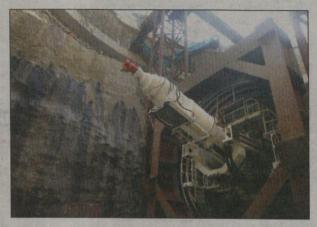
The machine was lowered into the shaft on Sept 21 and after most parts were assembled, it began tunnelling. Janak Rathod
