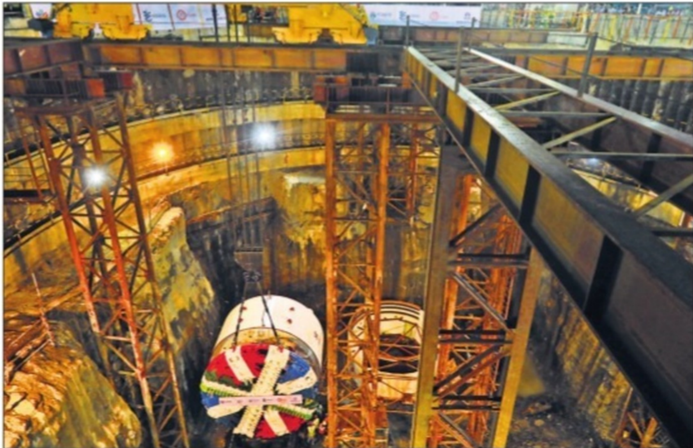
The cutterhead of the tunnel boring machine being lowered into the Nayanagar shaft in Mahim Thursday. (Left) CM Devendra Fadnavis at the site. Nirmal Harindran
