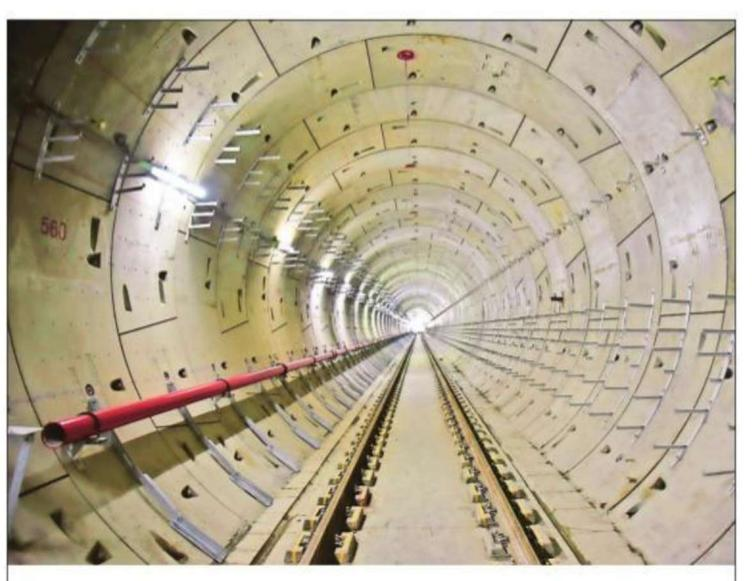
The tunnel boring machine, Tansa 1, completed its most challenging drive of 837 m from Mahalaxmi Metro Station to Mumbai Central Metro Station upline in 243 days, using 558 concrete rings. Express
