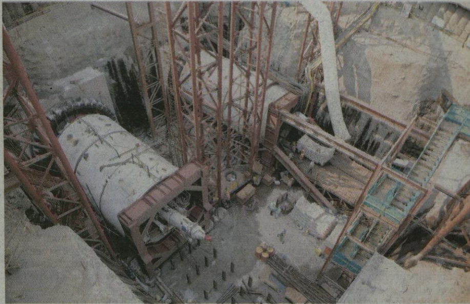
Digging away: The tunnel boring machine started operations at the launching shaft in Naya Nagar, Mahim, on Friday. ■ VIJAY BATE
