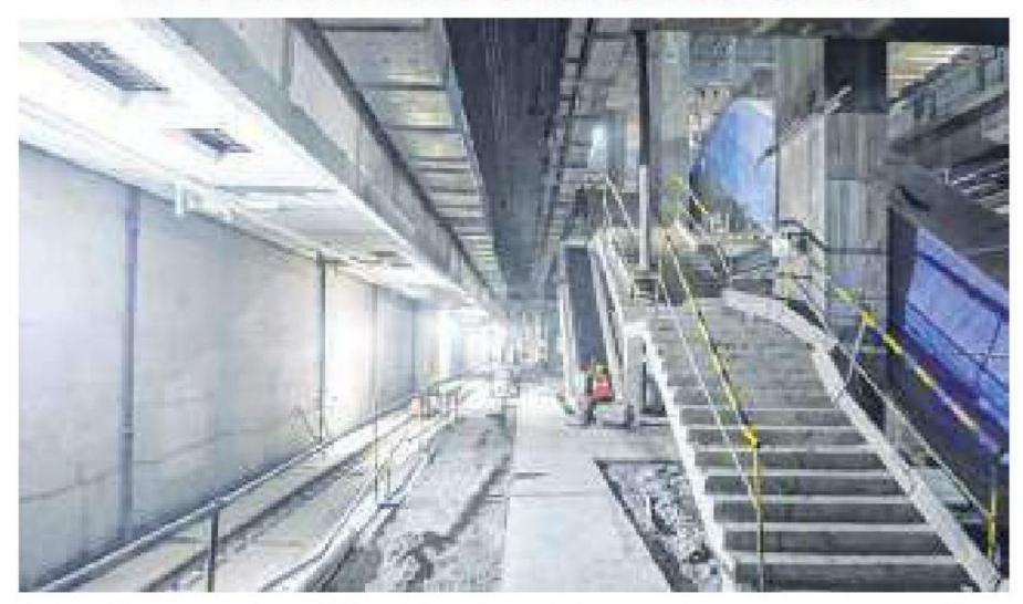
A view of the Dharavi Metro Station, which is being built in one of the most dense areas of the world. Currently road restoration, structural and architectural finishing works, and entry and exit points are in progress. Overall 89.2% of civil and 54.4% of systems works is completed.
