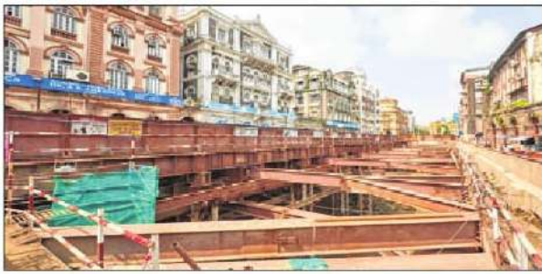
A view of the Metro 3 site near Fountain in south Mumbai
