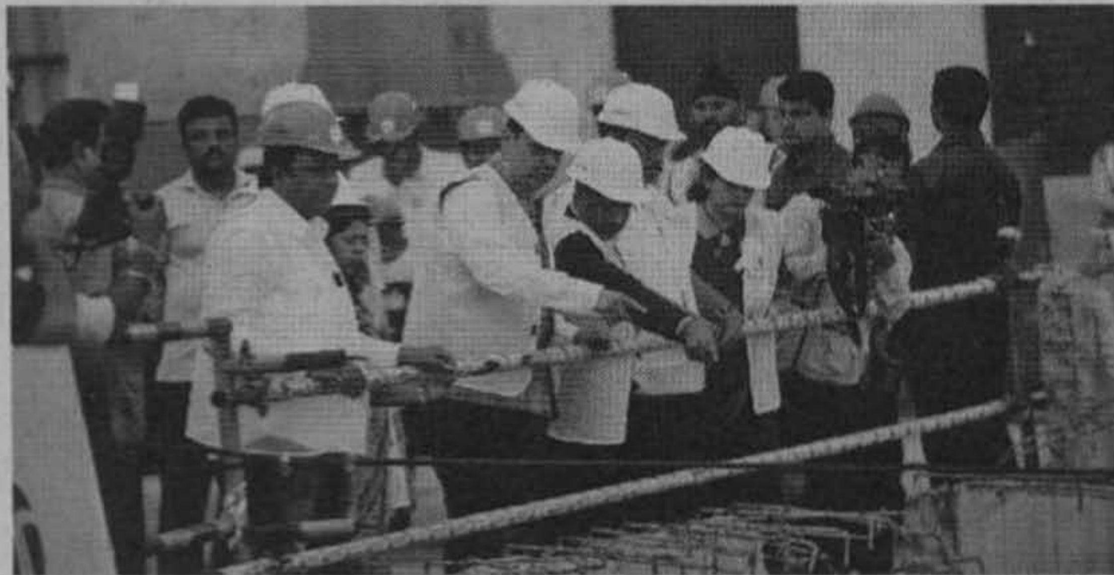
The chief minister at the lowering of the tunnel boring machine event.
