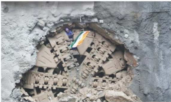
Wainganga 2 TBM breakthrough at SEEPZ.
