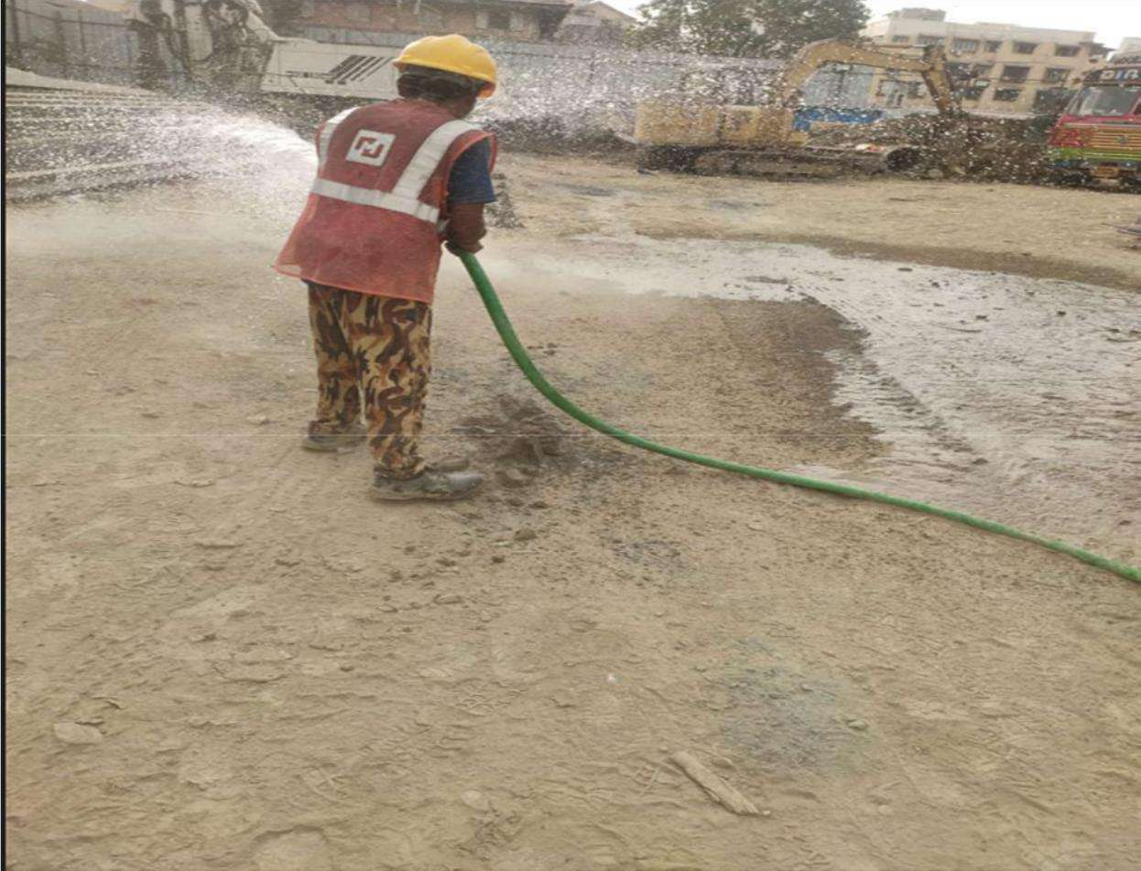
Sprinkling of water to control dust emission
