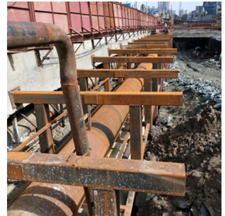
Supporting of 1800 mm Ø GFRP Pipe along with 900 mm Ø SWD at Acharya Atrre Chowk Station
