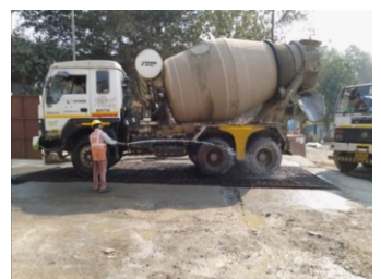
Step 6: Treated water is being used for gardening, road cleaning, dust control and vehicle wheel wash purpose.
