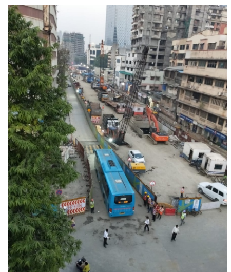
Concrete deck at Shitladevi Station
