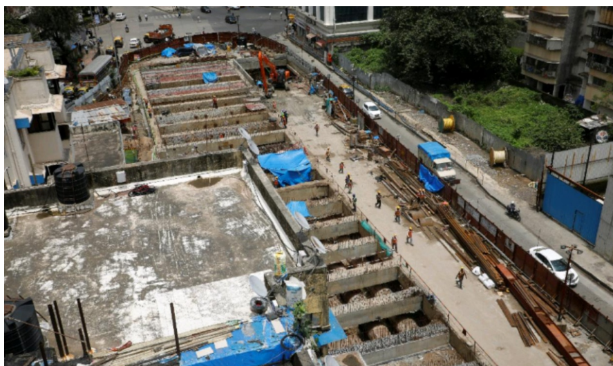
Concrete deck at Dadar Metro Station
