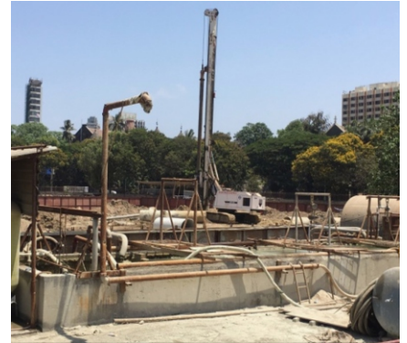
Step 3: After primary treatment, the treated water pumped from shaft sedimentation tank to surface sedimentation tank for further removal of suspended solids.
