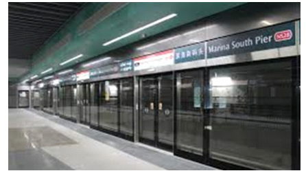
Platform Screen Doors (PSD)
