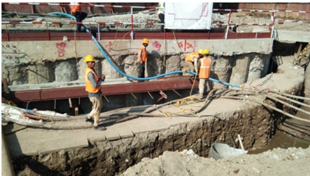
Step-1: Exposing of existing oil filled cables
