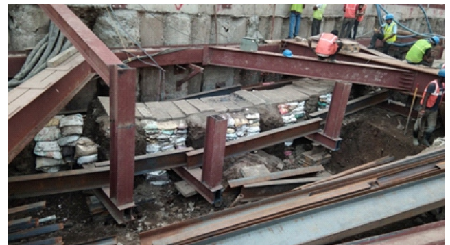
Step-2: Inserting bottom supporting member below the cables in staggered manner and supporting the same to secant pile wall.
