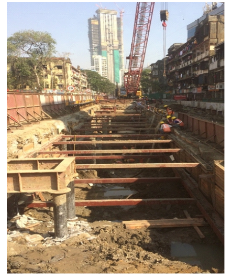
Step-1 Excavating Trench and side supporting
