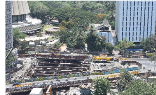
Steel Decks at Vidhan Bhavan Station
