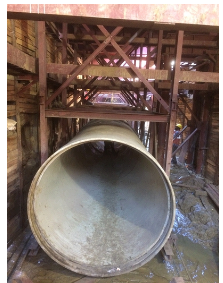
Step-3 Bottom supporting Cradle hung from Traffic decking
