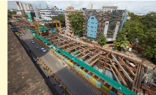
Steel Deck at Churchgate Metro Station
