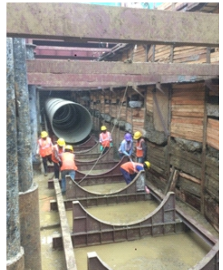
Step-2 Placing of GFRP Pipe above bottom supporting cradle beam
