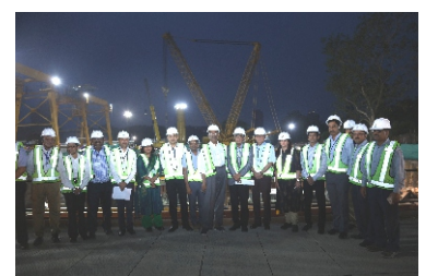
TBM Lowering at Azad Maidan
