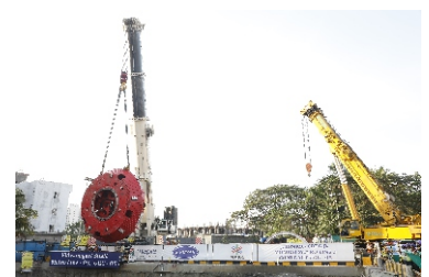
TBM Lowering at Vidyanagri
