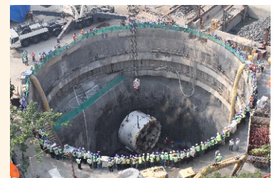
TBM Lowering at Pali Ground
