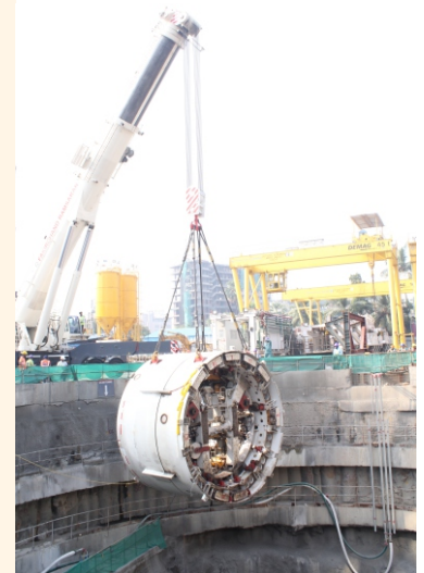
TBM Lowering at Pali Ground
