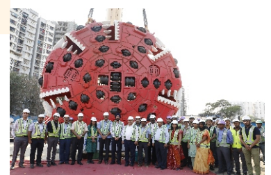
TBM Lowering at Vidyanagri
