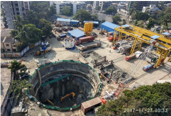
STEC TBM different parts received and successfully unloaded at Pali Ground
