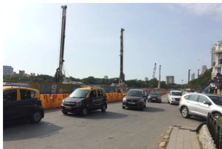
Station Work in Progress
