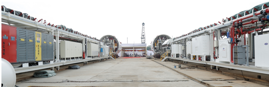
Rear view of TBM with support gantries
