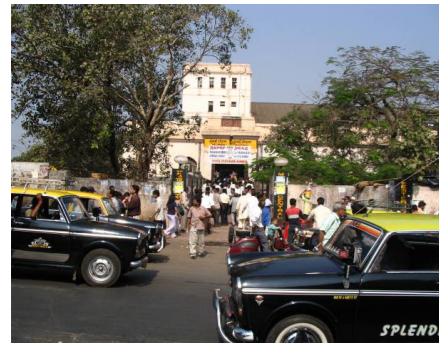
View of Station from Bellasis Bridge
