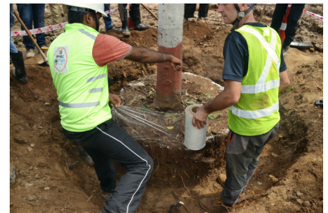
Packing of root-ball
