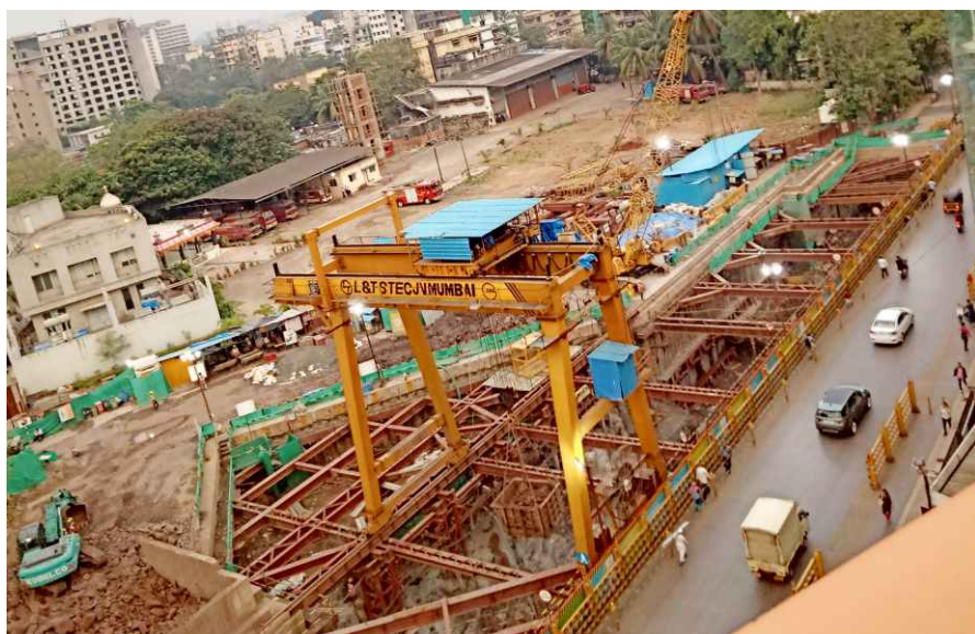
Marol Naka Station Work is in Progress
