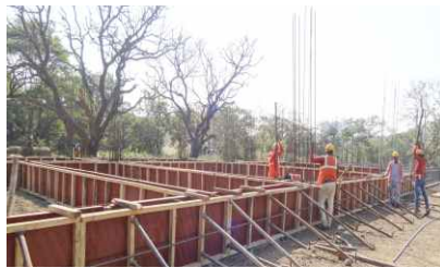
Work Shop at Depot
