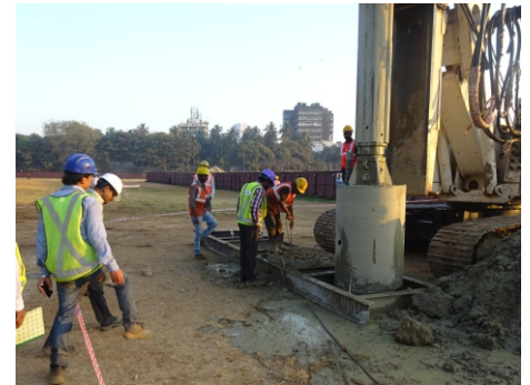
Secant Piling in CST
