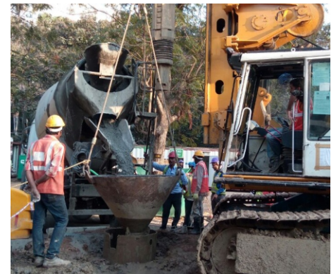
Piling at Cuffe Parade
