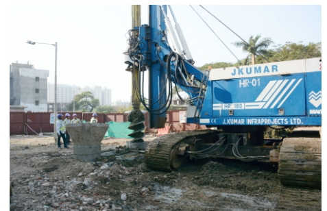
Secant Piling at Vidyanaigari Station
