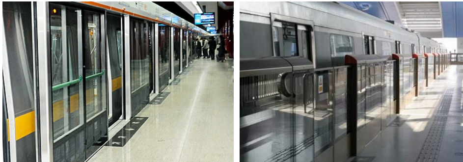
Two types of doors : Platform Screen Door and Platform Edge Door
