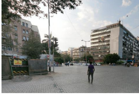
Churchgate Suburban Station, Metro construction work in progress
