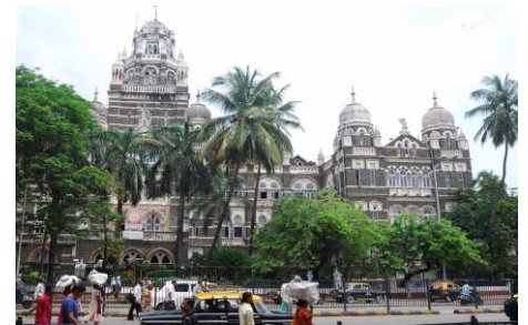
Western Railway Headquarters, Churchgate Source: www.wikiwand.com
