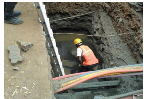
Excavation for utility diversion at Science Museum
