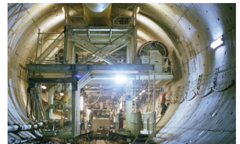
Completed Metro Tunnel Lining
