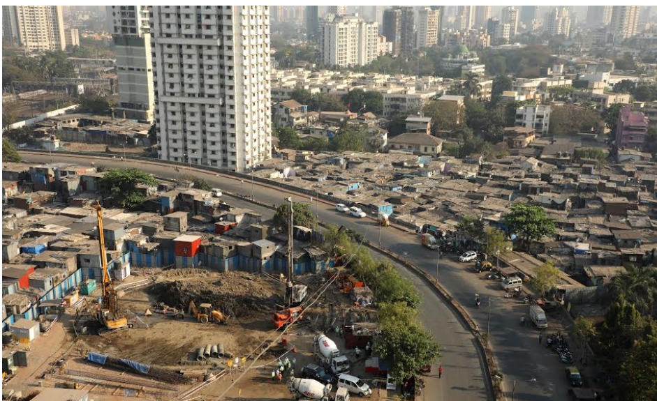
TBM launching shaft construction in progress at Nayanagar
