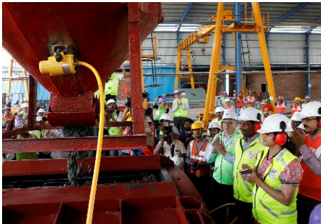
Pouring of first segment ring at Wadala casting yard
