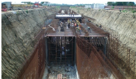
Cut & Cover Tunneling in Delhi International Airport Area (Phase 3)
