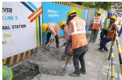
Cleaning of Storm Water Drains
