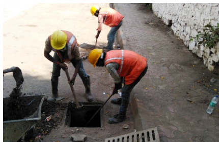
Drain Chamber Cleaning
