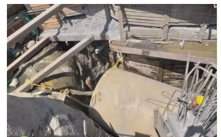
Chamber Connection work at Grant Road Station
