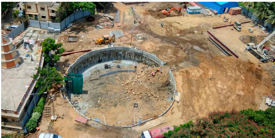
Secant Pile - L&T UGC-07, Pali Ground, SEEPZ
