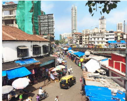
Frere Bridge as seen from Grant Road skywalk
