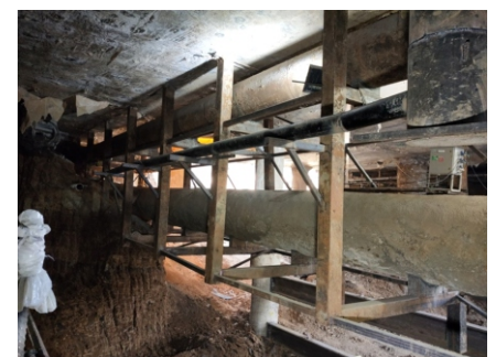
Existing Sewer Line is supported at Worli Station
