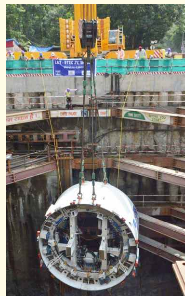
Two TBMs have been lowered and are getting assembled for tunneling.
