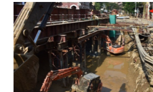
Utilities at Hutatma Chowk Station
