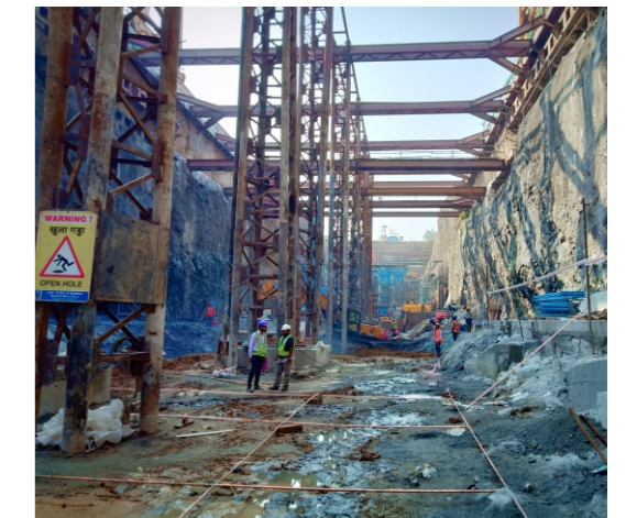
MIDC station work is in progress
