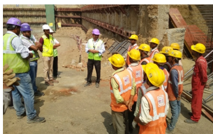
Quality Team Training for good workmanship at Metro-3 Site
