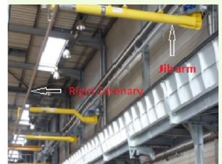
(b) Retracted Position (For overhead maintenance of a Train)
