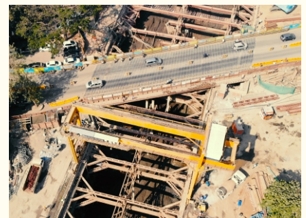
An elaborate steel deck installed at Vidhan Bhavan metro station so that traffic can move swiftly along with taking place underground Metro-3 work.
