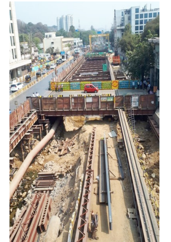
SEEPZ Station work is in progress
