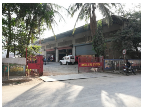
Marol Fire Station
