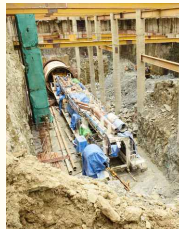
Tansa-1 TBM Assembly
