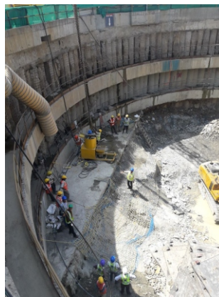
Launching Shaft, Pali Ground
