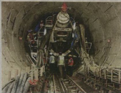
The TBM at Naya Nagar. PIC/SURESH KARKERA
