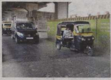
Temporary barricades installed on roads for Metro Line 3 work
