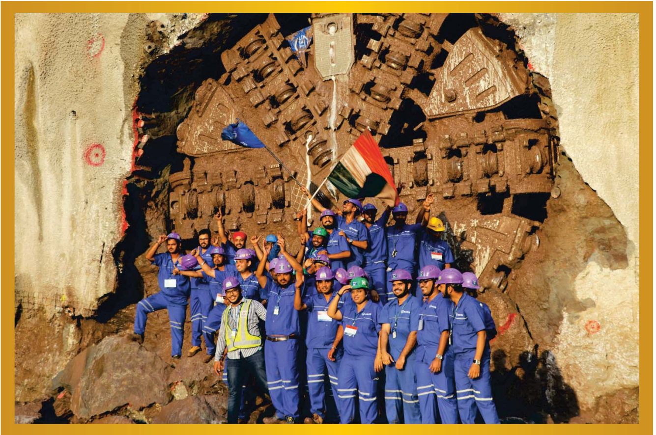
First TBM Breakthrough of Mumbai Metro - 3
