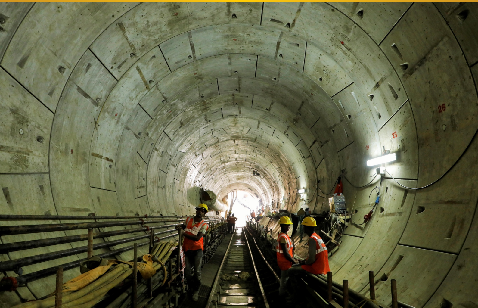
Tunnelling in progress
