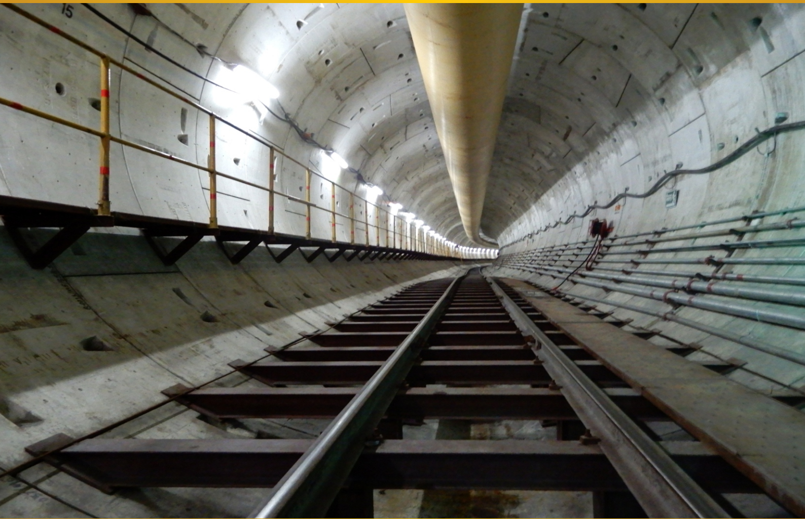
Tunnelling in progress
