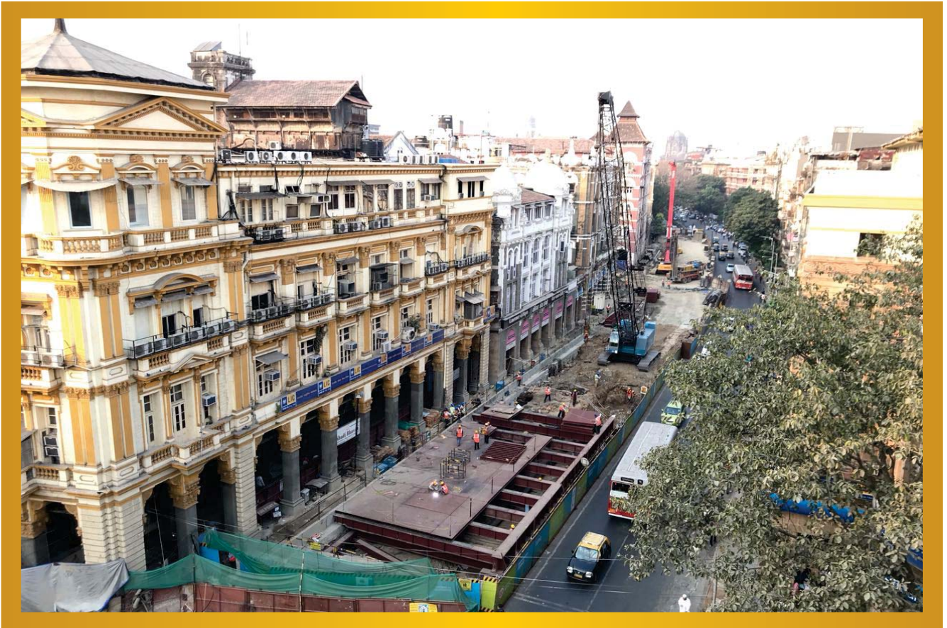
Work in Progress at Hutatma Chowk
