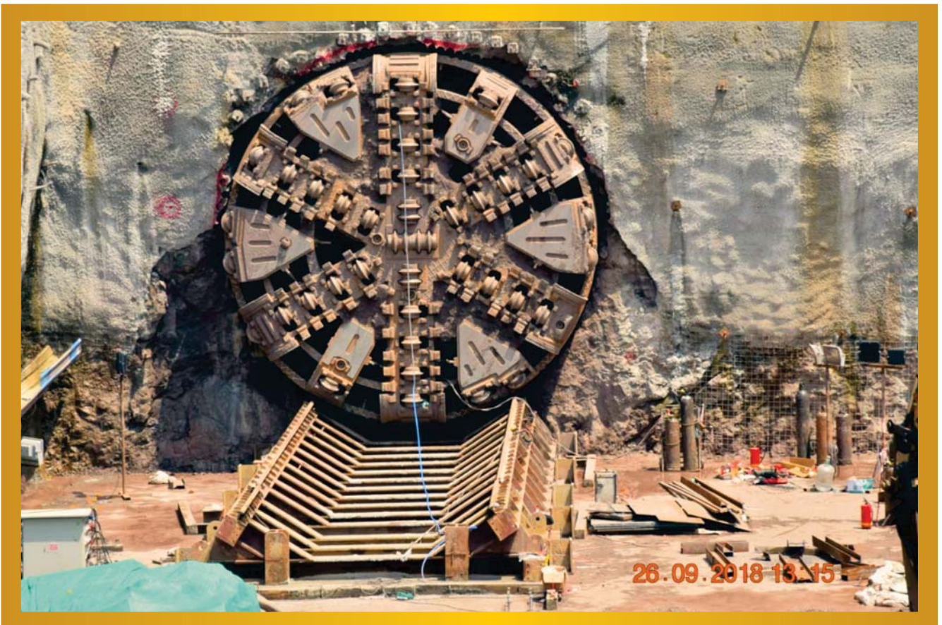
First TBM Breakthrough of Mumbai Metro - 3
