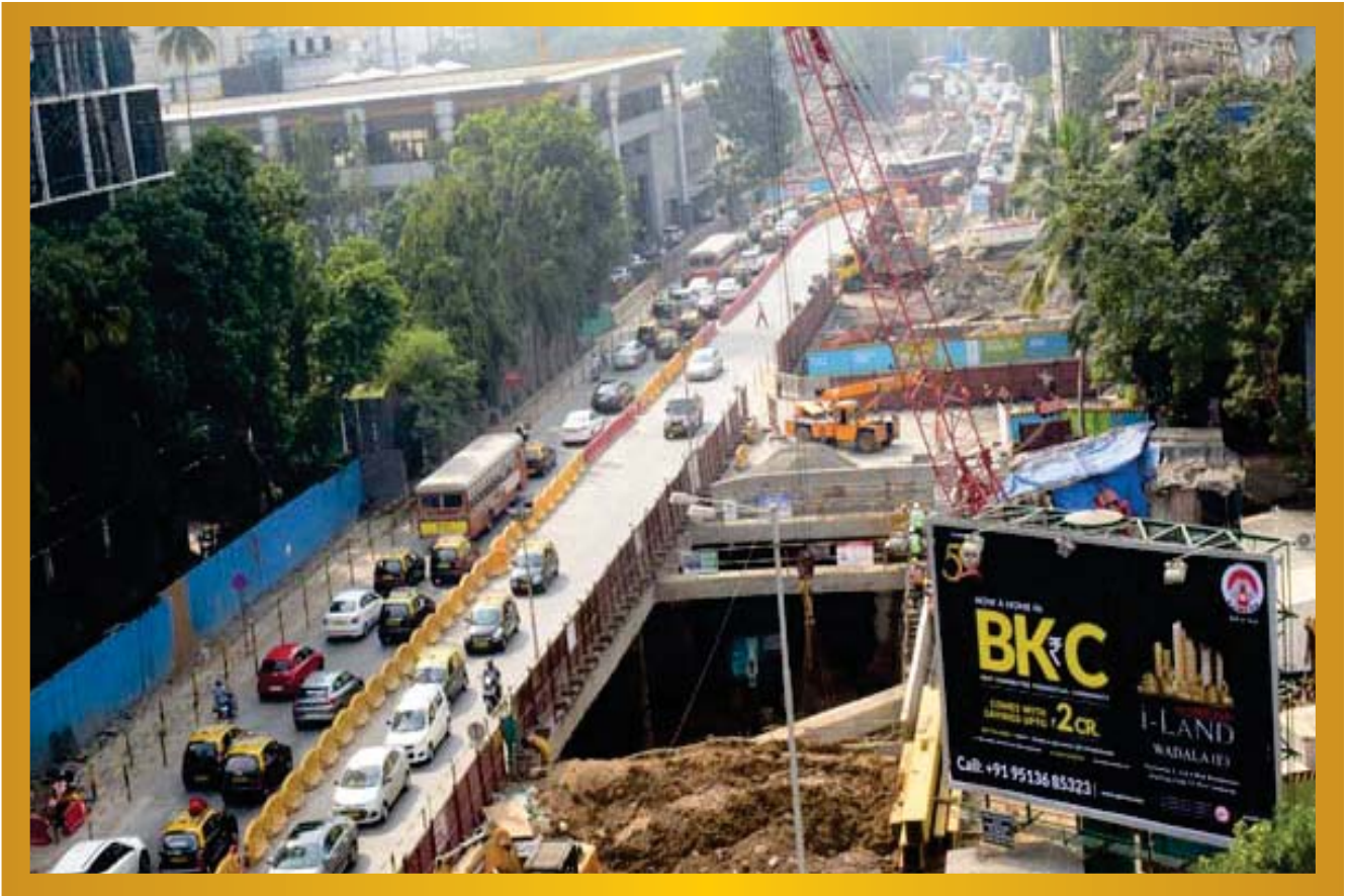
Bird's Eye View of Work in progress at Worli
