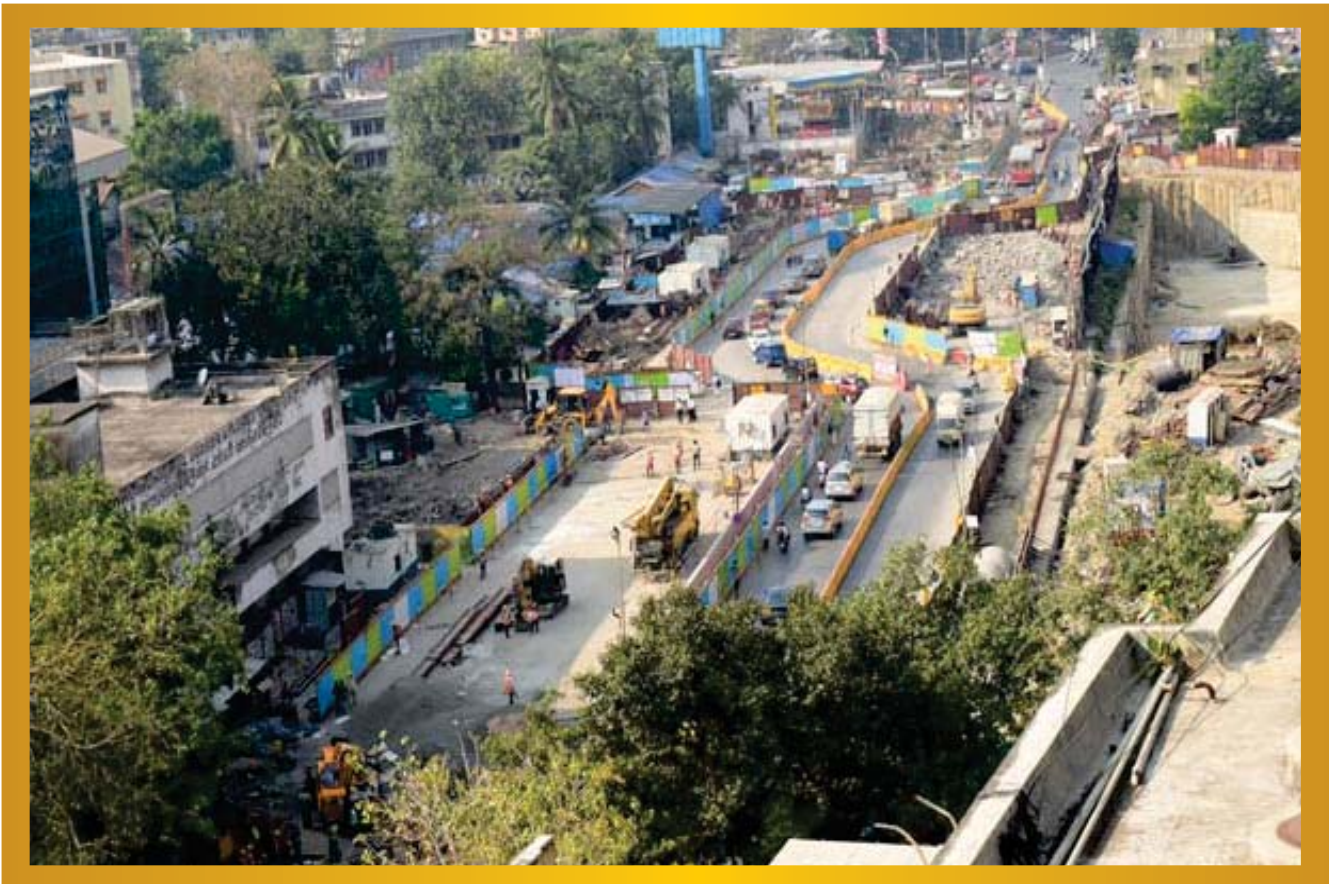
Bird's Eye View of Work in progress at Acharya Attre Chowk
