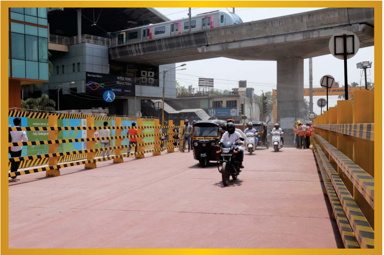
Steel Decking Work at Marol-Maroshi road at Marol Naka station
