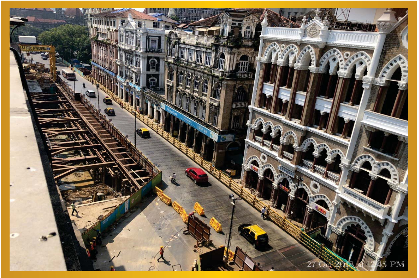
Bird Eye View of Work in progress at Hutatma Chowk..
