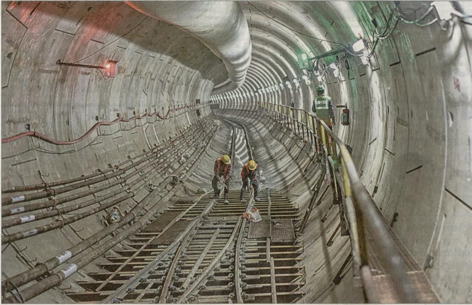
▪ (Left) Colaba to Seepz via Bandra within minutes? It doesn't come easy. It has been almost a year since the work on the tunnel at Nayanagar in Mahim started. The 51-km tunneling will need 2.8 lakh separate segments. Ditto for the Airport Metro (above). Building a tunnel from Pali Ground in Marol to the T2 international airport took almost eight months. End result? A 1.26km tunnel and 1.5 lakh cubic meters of muck.
