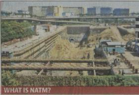
■ The New Austrian Tunnelling Method (NATM) is a modern tunnelling method appropriate for congested spaces.
