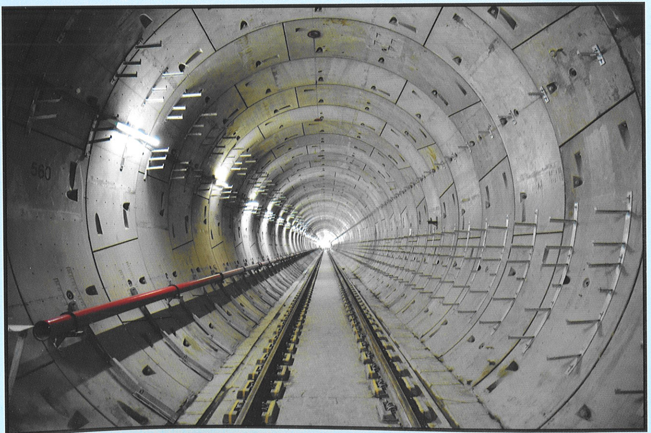
Completed Tunnel along with tracks of Metro-3
