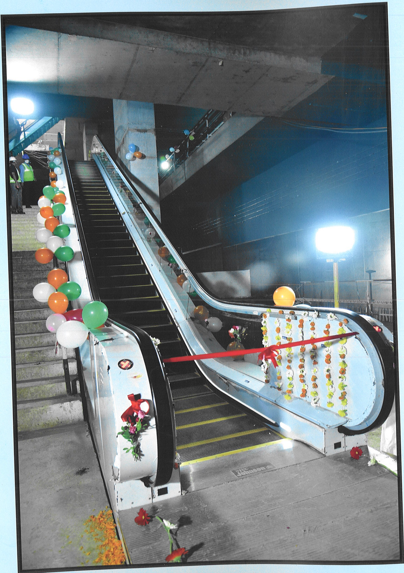
First escalator of Siddhivinayak Metro station set up
