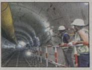
MMRCL, by using the New Austrian Tunnelling Method (NATM) in which the traditional excavators are being used. From Monday work for casting of permanent lining started.
