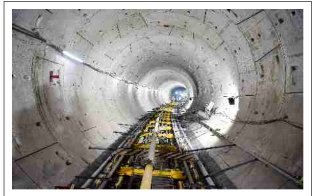
Work in Progress at metro 3 - Tunnel along with tracks
