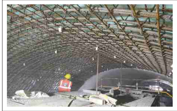
Glimpses of NATM- Overt work at Cuffe Parade metro station
