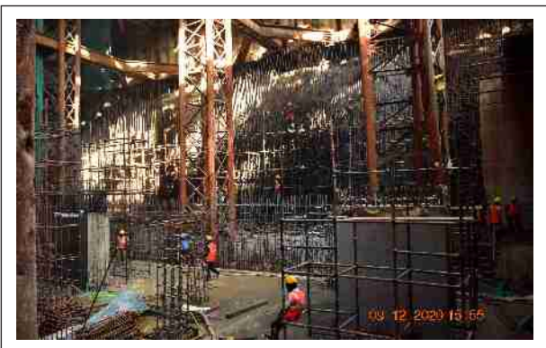
wall rebar work in progress at SMC
