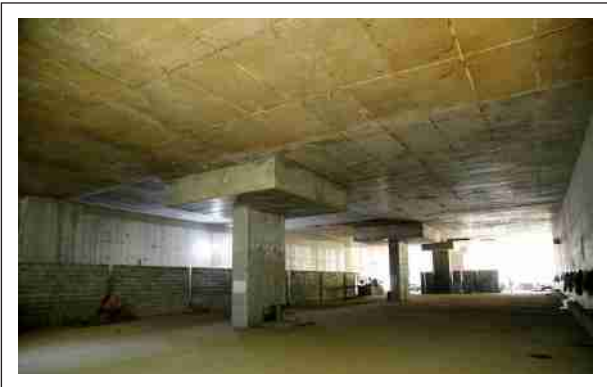
Work in Progress at Siddhivinayak Station
