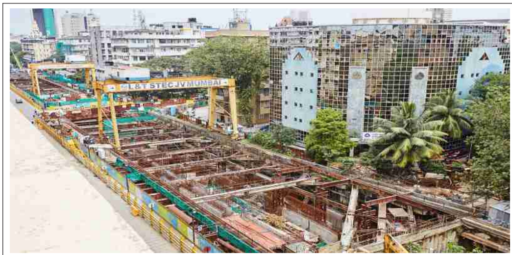
Aerial View of Churchgate Metro Station
