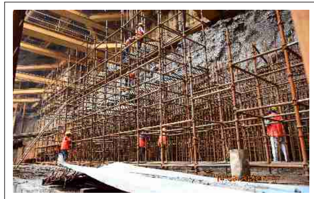
Side Walls work in progress at Mumbai Central
