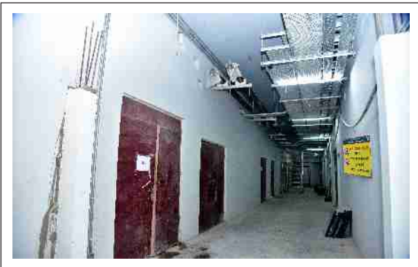
Work in Progress at Seepz
