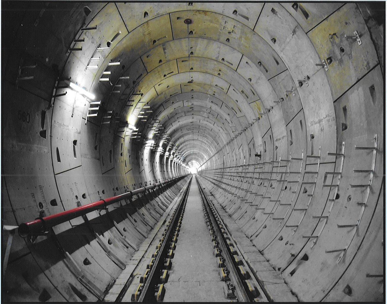
Completed Tunnel along with tracks of Metro-3
