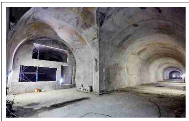
Glimpses of Cross Over work at Cuffe Parade Metro station
