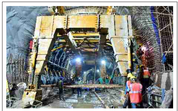
NATM Work in progress at T2 Metro Station
