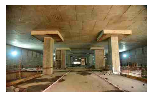
Ongoing Station interior work at BKC station
