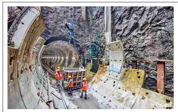
Work In Progress at Churchgate Metro Station
