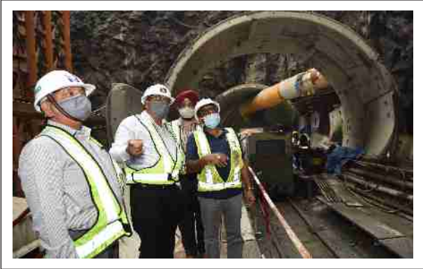
Site visit of GM, Central Railway at Hutatma Metro station
