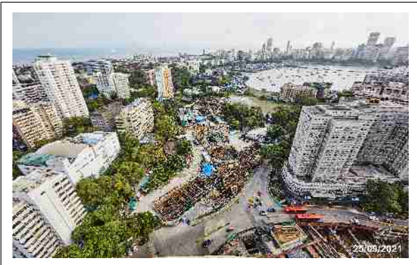
Aerial View of Work in Progress at Vidhan Bhavan Metro Station
