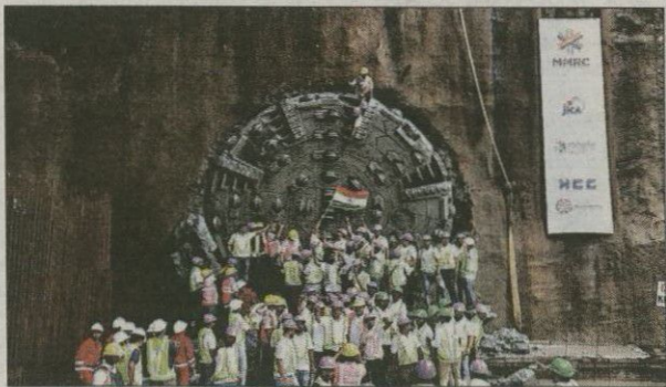
Tunnel boring machine Vaitarna
