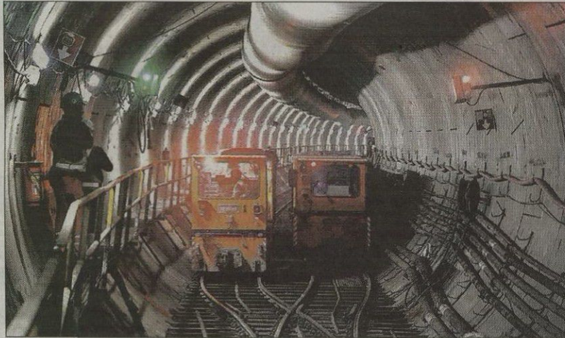
Construction work for Metro-3 corridor underway at Mahim's Naya Nagar
