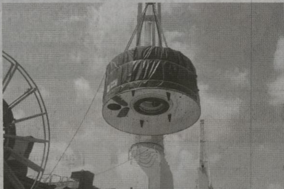
The TBM will function from this month itself.
